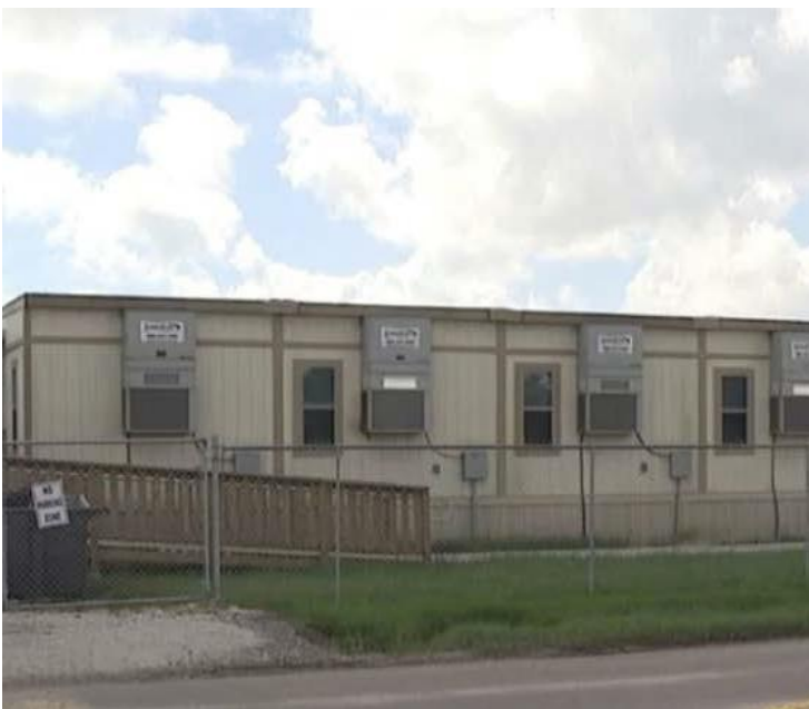
A school district in East Texas used DRS' MVP Program to source and install temporary classrooms for 1,100 students within 10 weeks of the flood event, getting students back into classrooms quickly and safely.
