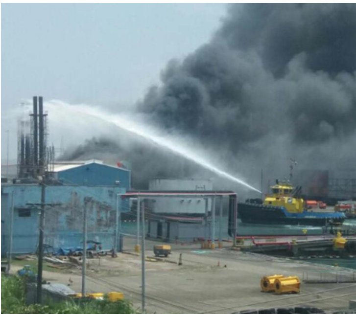
After a gas leak caused an explosion, a power generation company in Panama used DRS' MVP Program to source and install a replacement barge reducing their period of interruption to less than a year.
